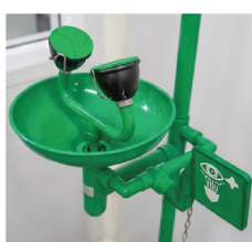
Eye wash station
